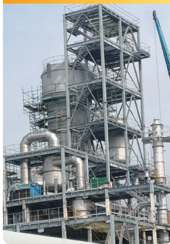
▲ 石化廠塔槽安裝 Petrochemical Tower Installation
